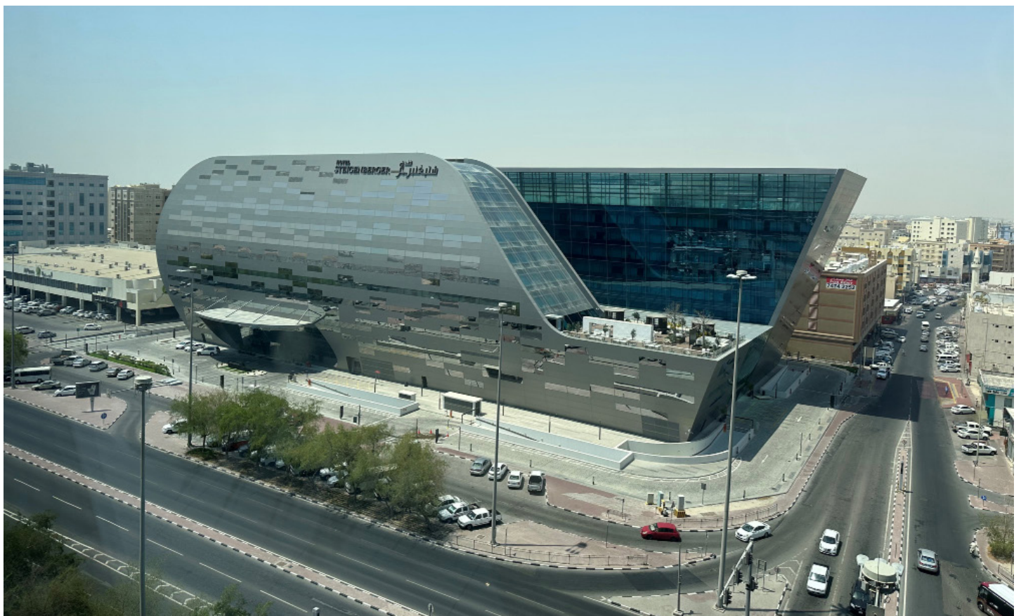
Steigenberger Hotel - Doha, Qatar
