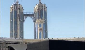
Zones N1 and N6A are connected via a sky bridge used as a praying area. The bridge is linked to the two twin towers at the 37<sup>th</sup>, 38<sup>th</sup>, and 40th floors; with an elevation of 40 meters length, and at a height of 165 meters above the ground.
