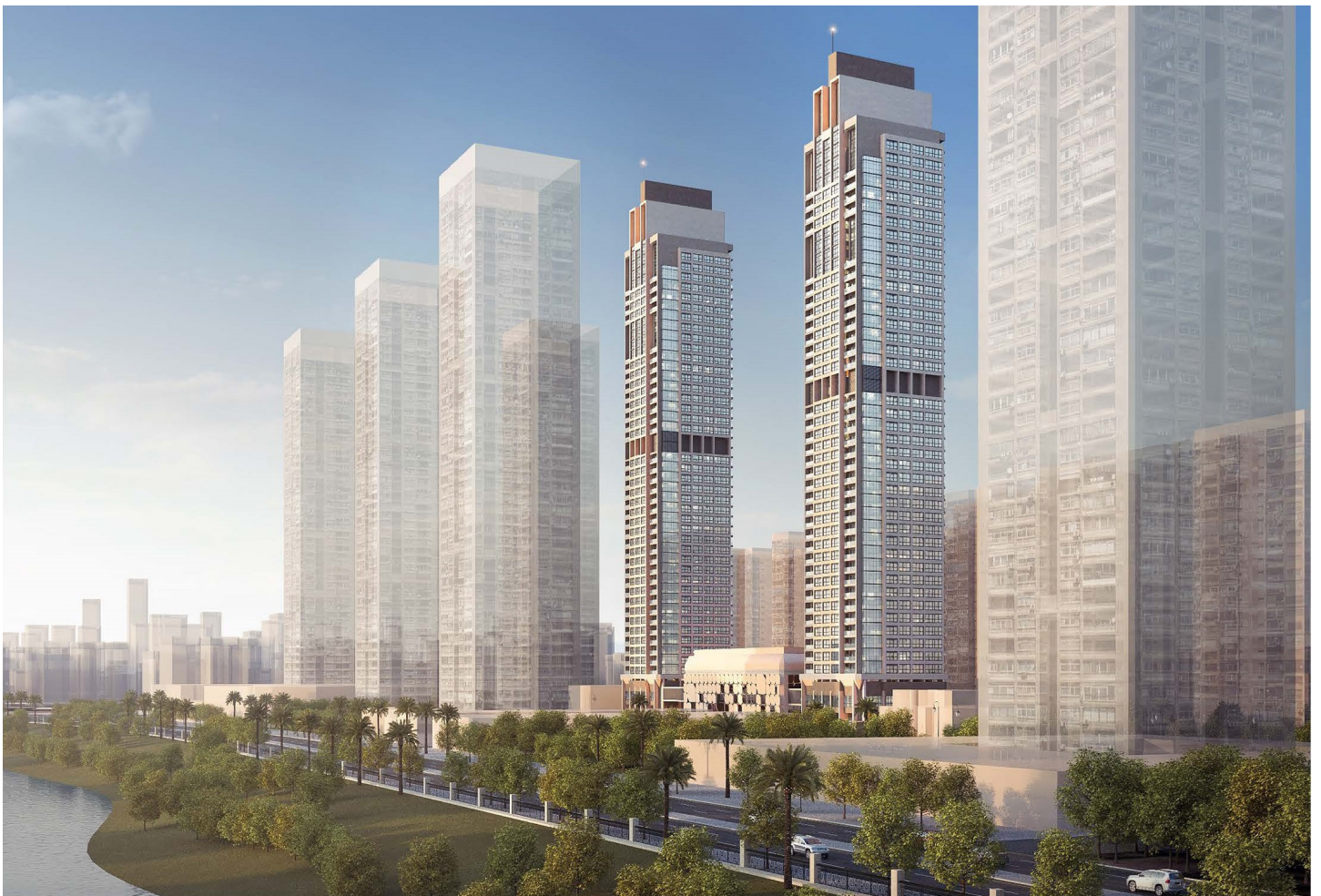
Two Residential Towers (A5 & A3) in Maadi
